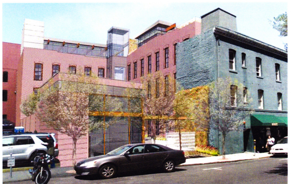
MUSTO BUILD-OUT —A 4th floor addition has been reduced in scale from previously proposed projects and has been set back from the existing perimeter walls in order to preserve the massing of the original building, according to the Project Manager.
